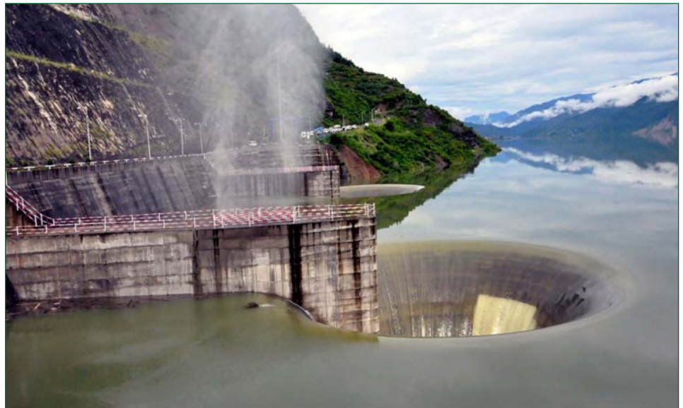
Tehri Right Bank Shaft Spillway (Morning Glory) in operation evacuating floods above the Full Reservoir Level
